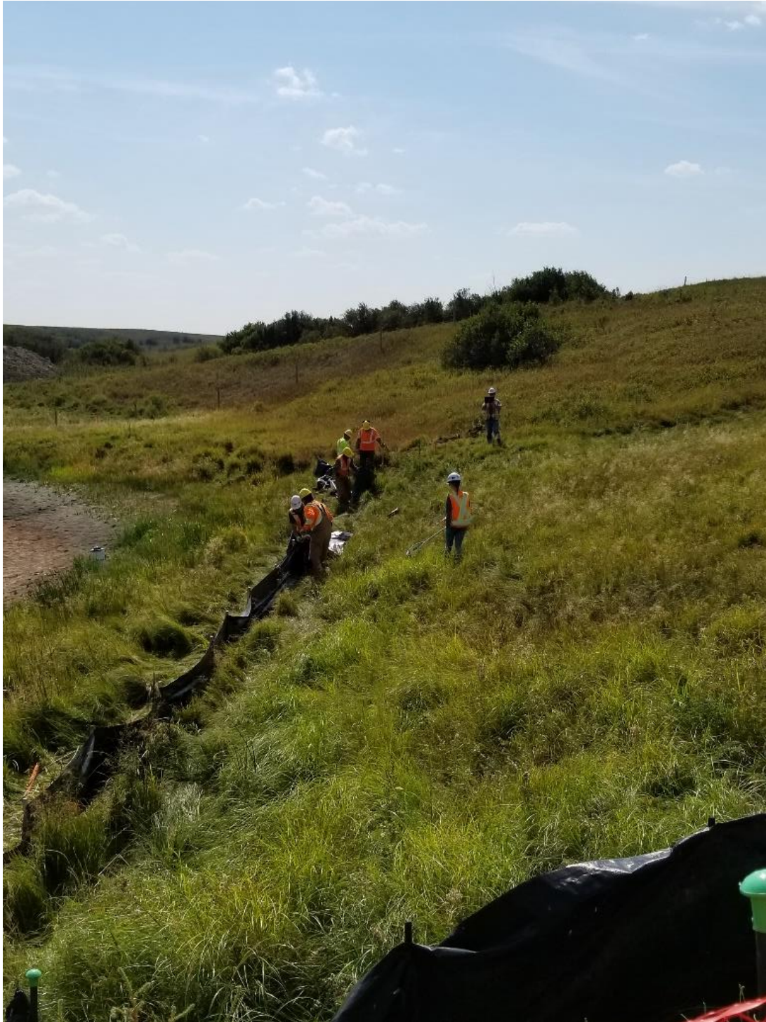
Installation of Silt fence to keep out excess dirt as they begin stripping the topsoil.
